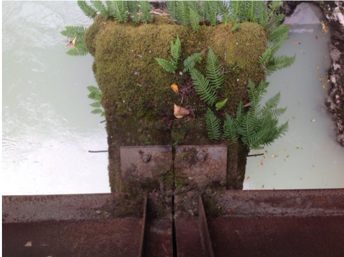
left span upstream pier bearing
