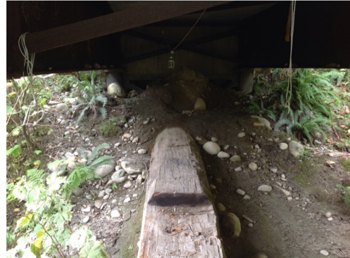
Right Bank Abutment when facing downstream
