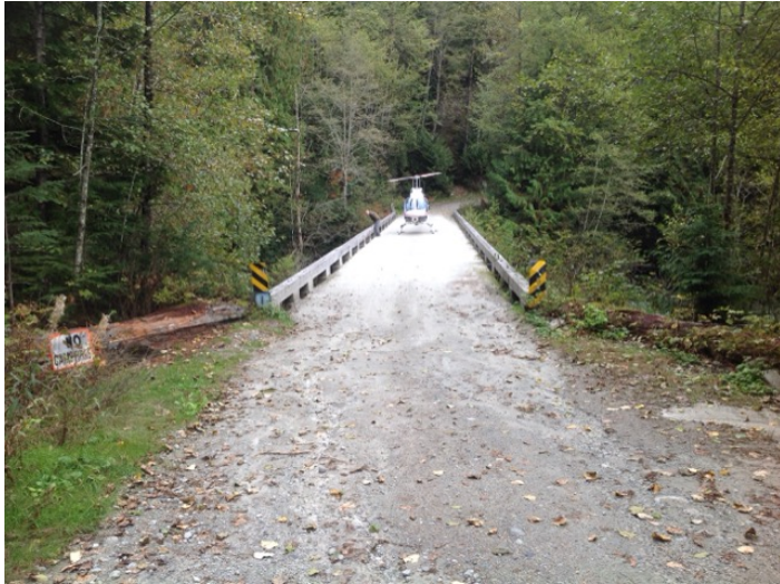
Approach from Right Bank when facing downstream
