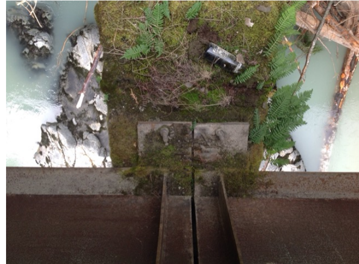
right span upstream pier bearing
