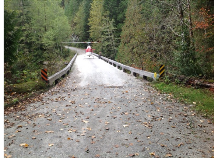
Left Bank Abutment when facing downstream
