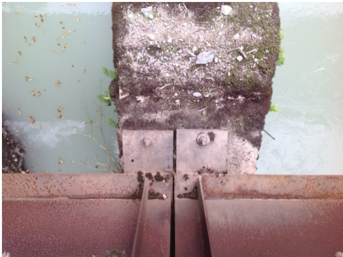
left span downstream pier bearing
