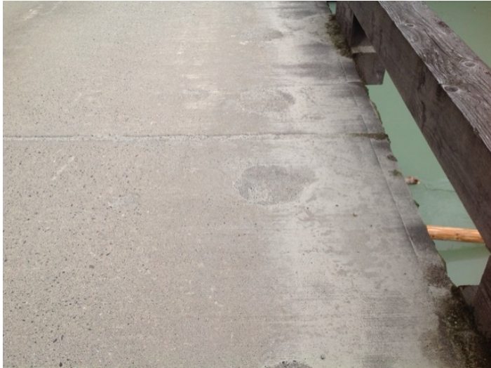
grout pockets - typical
