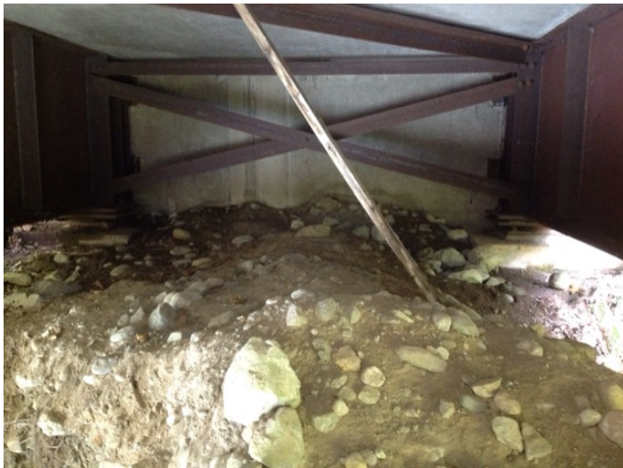
Left Bank Abutment when facing downstream
