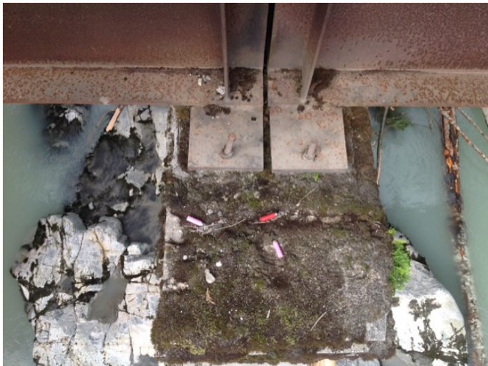
right span downstream pier bearing
